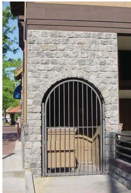
Utilities should be screened with landscaping
