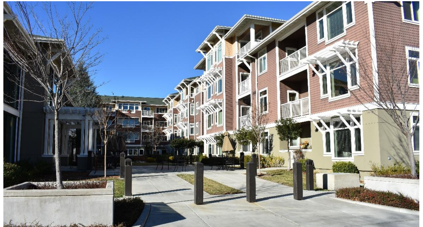
Figure 15 Shared Community Courtyard, Winters, California
