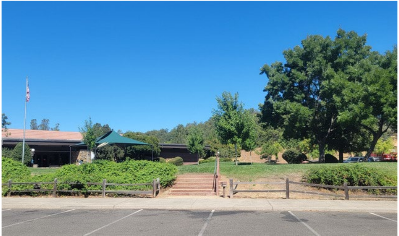
Existing site before construction
