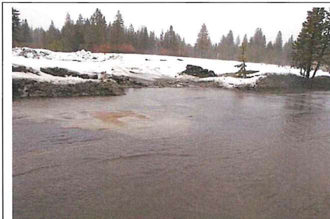
Pt #15: 02/08/2017 winter storm – Lot entrance
