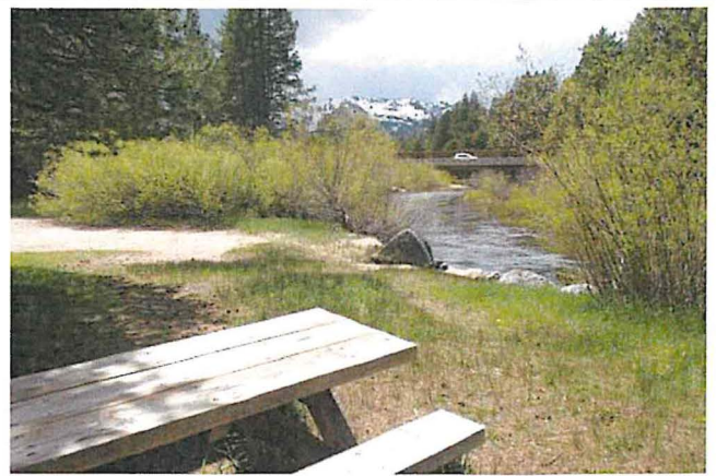
Photo Pt #8: looking west at Hwy 50 crossing
