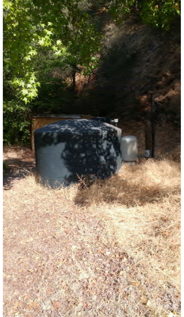
Photo 5 - Water Storage Tank
