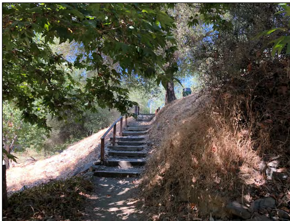
Photo 22: Staircase between gravel parking lot and lower terrace
