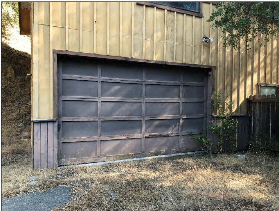
Photo 8: Garage on western half of house
