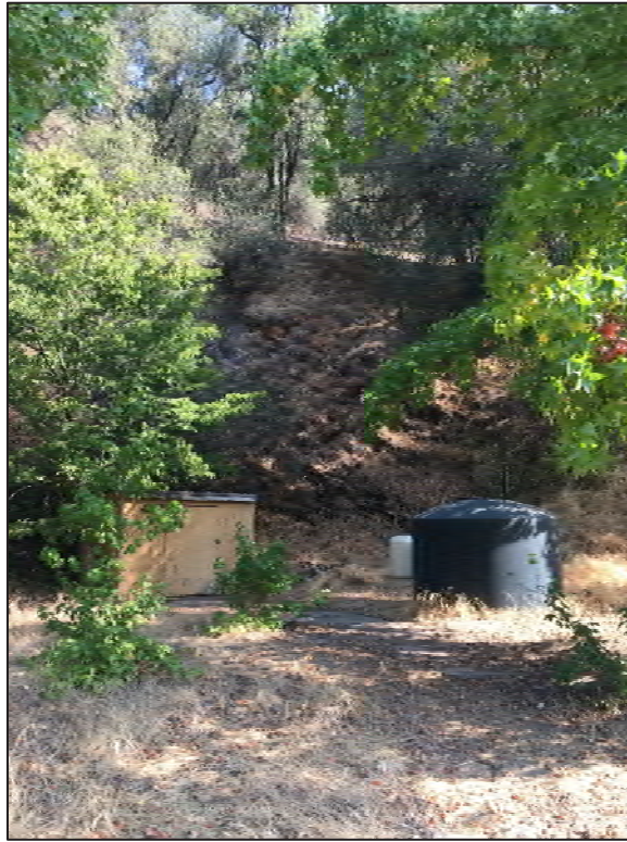
Photo 13: Water storage tank and shed
