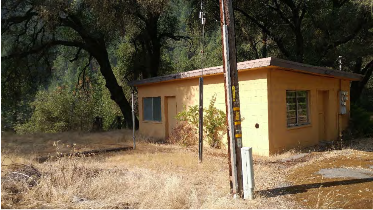
Photo 3 - Restroom Facility (septic tank assumed to be in this area)
