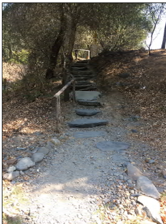
Photo 21: Staircase between gravel parking lot and lower terrace
