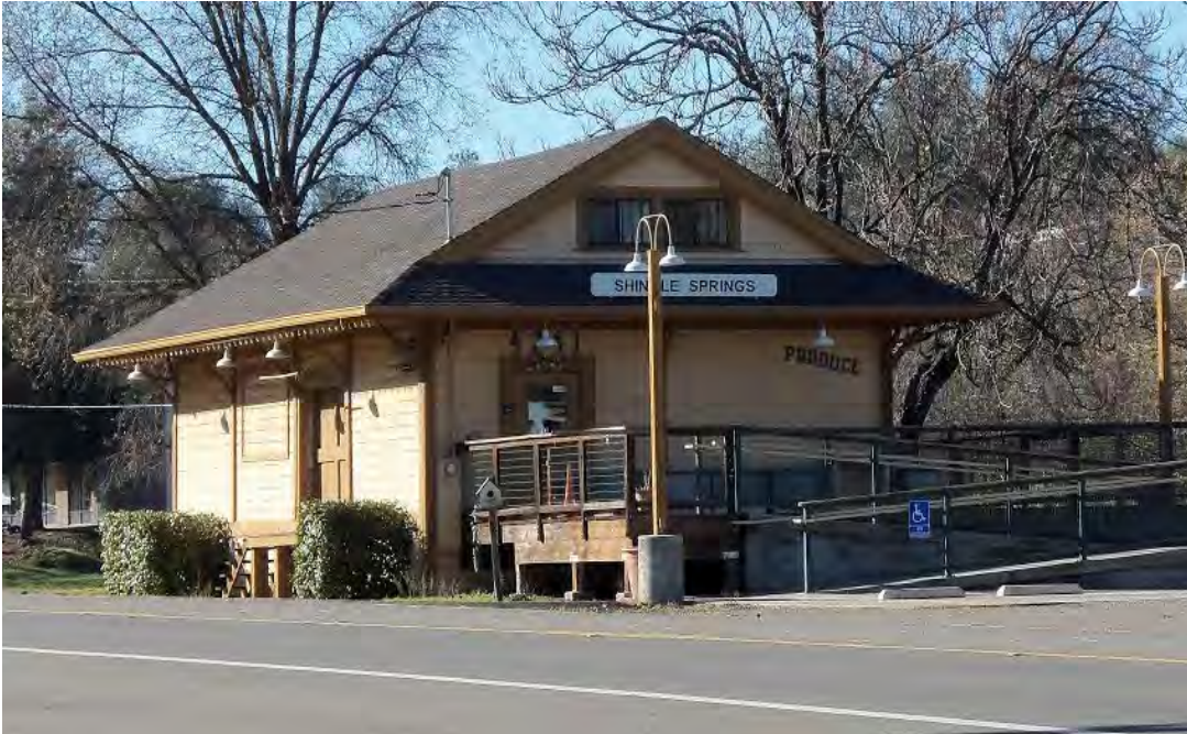
Figure 1: Shingle Springs Railroad Depot (single-story structure)
