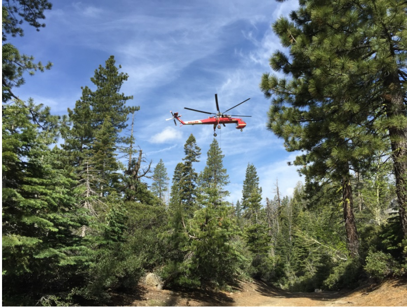
Rock drop between Ellis Creek and the FOTR Bridge.
