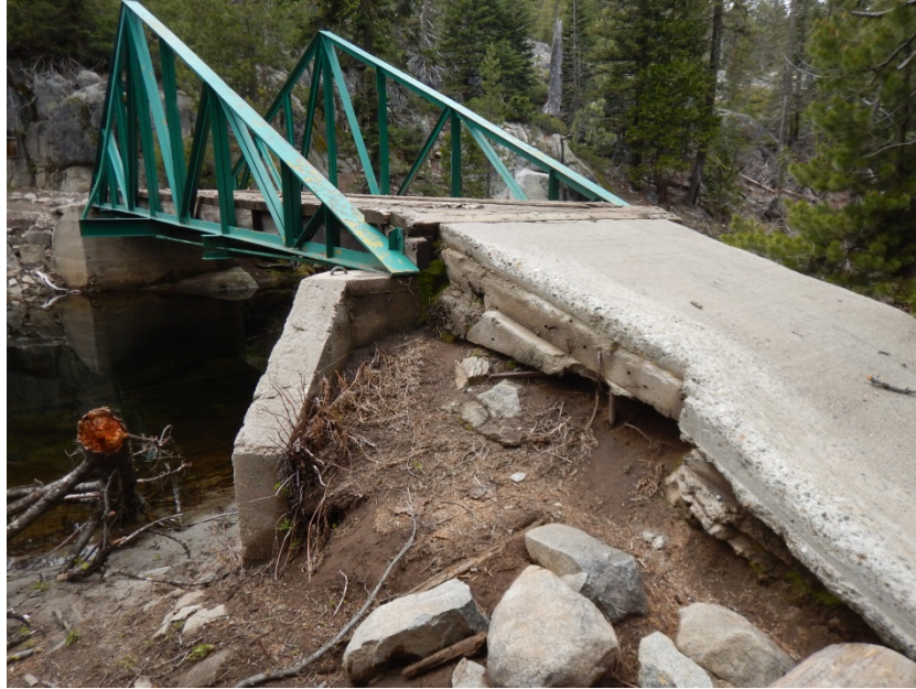
Old Bridge Abutment
