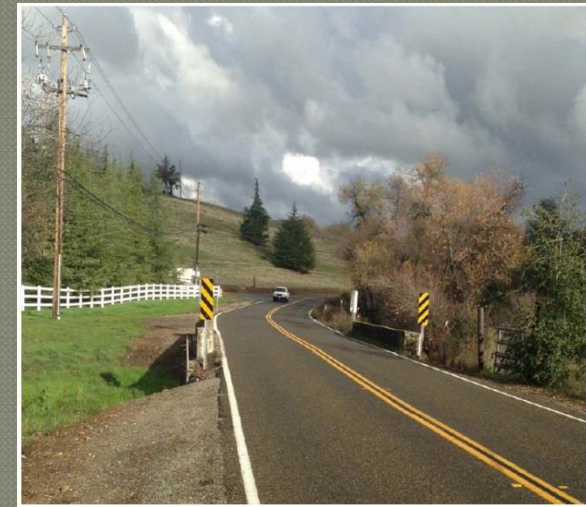
Green Valley Road at Mound Springs Creek Bridge
