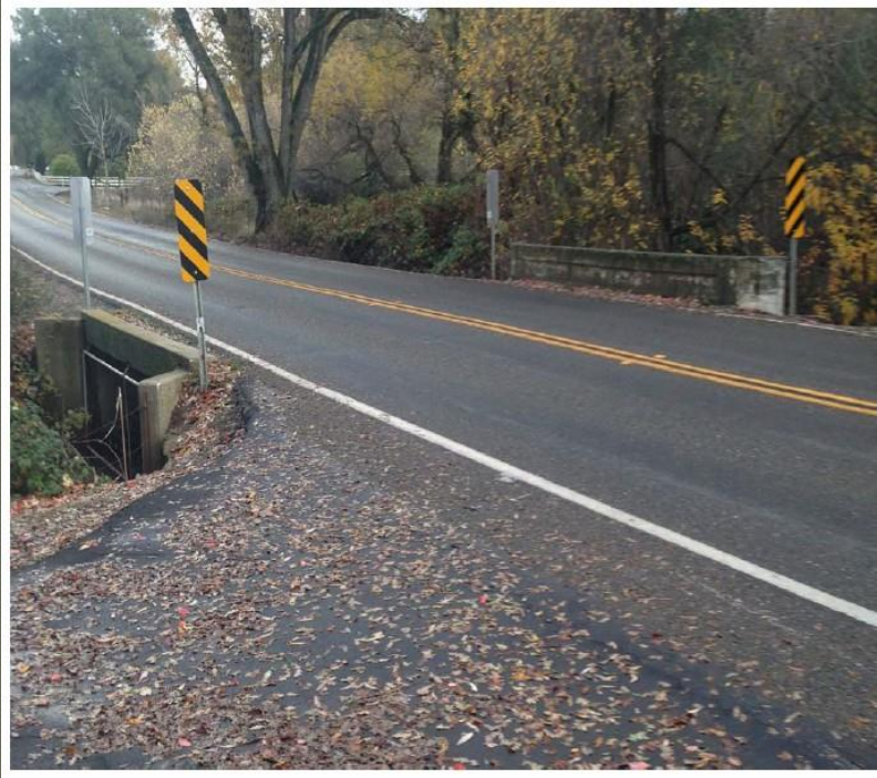
Green Valley Road at Indian Creek Bridge
