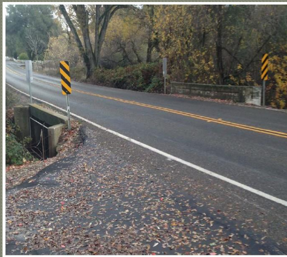
Green Valley Road at Indian Creek Bridge
