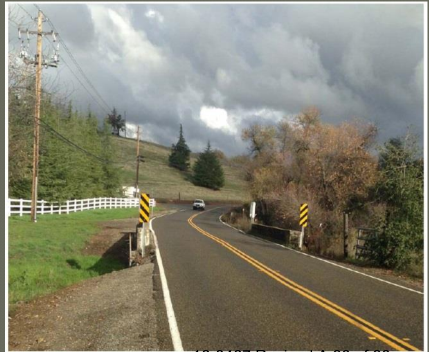
Green Valley Road at Mound Springs Creek Bridge
