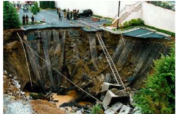
Collapses, such as the sudden formation of sinkholes, may destroy buildings, roads, and utilities.
