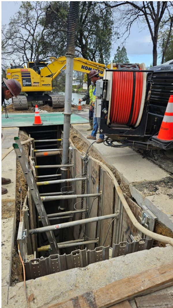
15' deep culvert excavation under Patterson Drive
