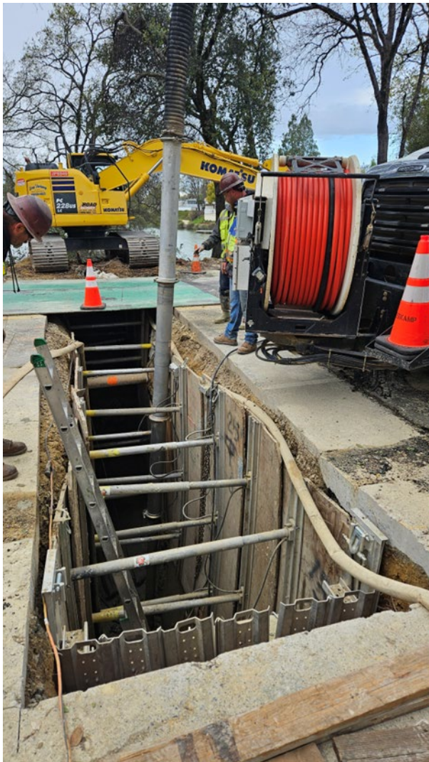
15' deep culvert excavation under Patterson Drive
