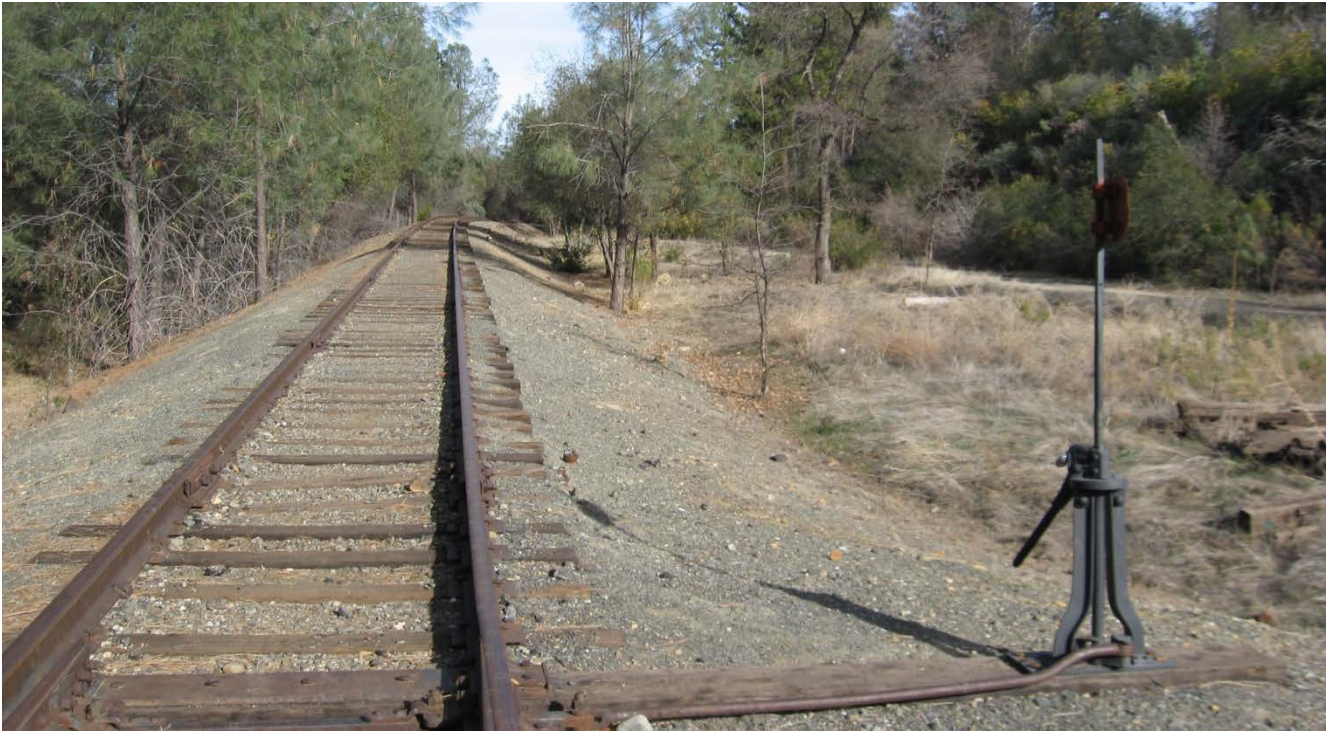
1 SPTC Right of Way, just west of Missouri Flat Road, looking northeast. Class 1 Trail would be built parallel to the existing railroad tracks to preserve the tracks.
