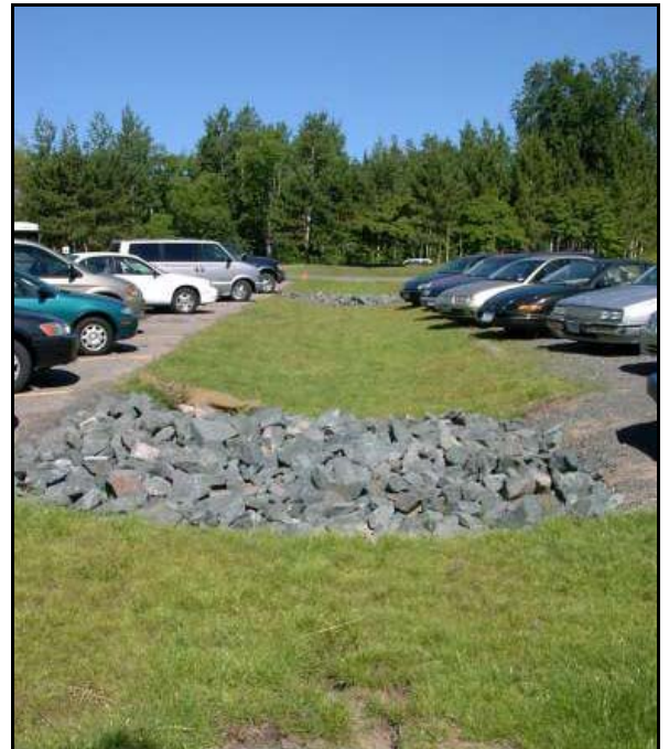
Grassy swale used to filter parking lot runoff
