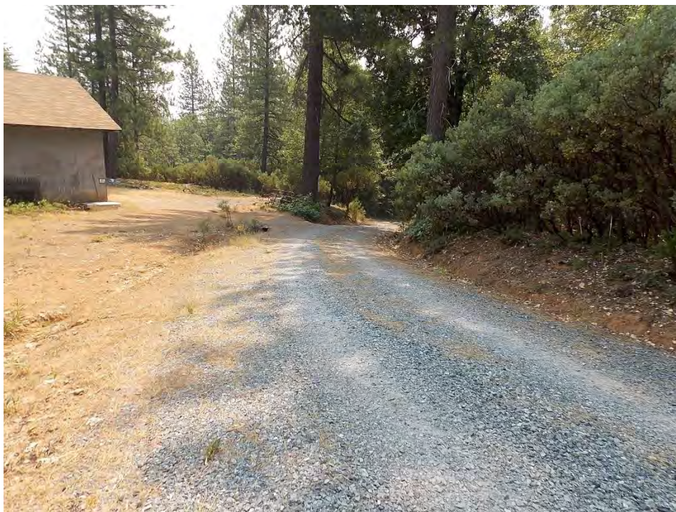
Photo 8: View from the south corner of the BSA showing the location where the proposed access road will tie into the existing road. 20 July 2017.
