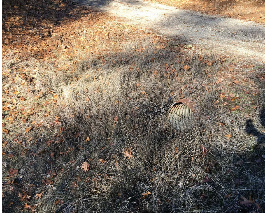
Photo 7. View looking northeast towards culvert inlet in the ephemeral channel. 6 December 2018.
