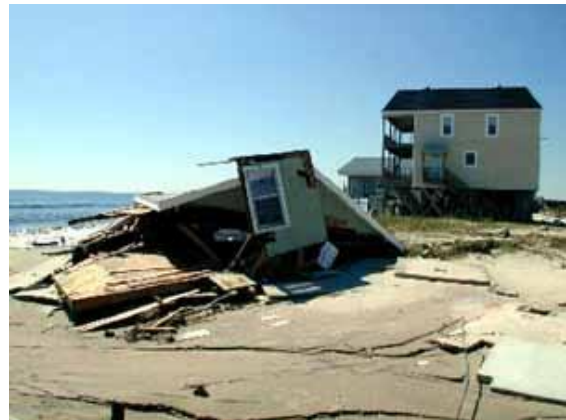
Hurricane Floyd brought a devastating 15 feet of storm surge that damaged or destroyed hundreds of houses along the ocean front of Long Beach on Oak Island, North Carolina in September 1999. A prime example of successful hazard mitigation, the elevated home (right) survived while the older, ground-level block foundation of the home on the left was crushed.
