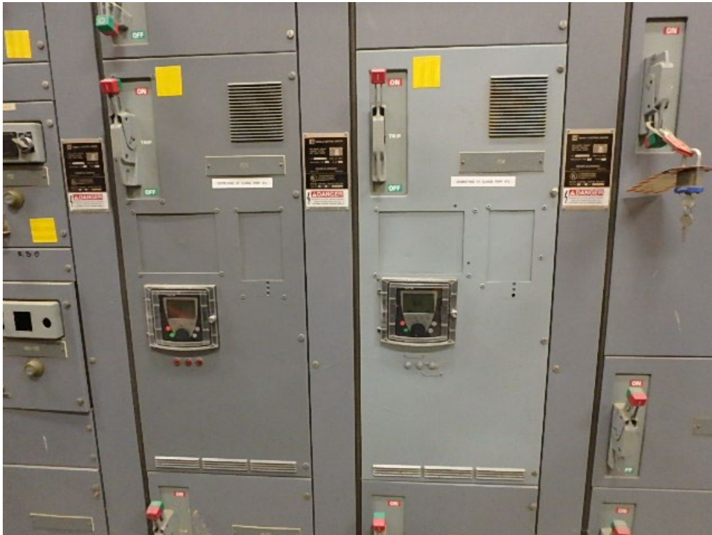
Centrifuge Feed Pump VFD Example
