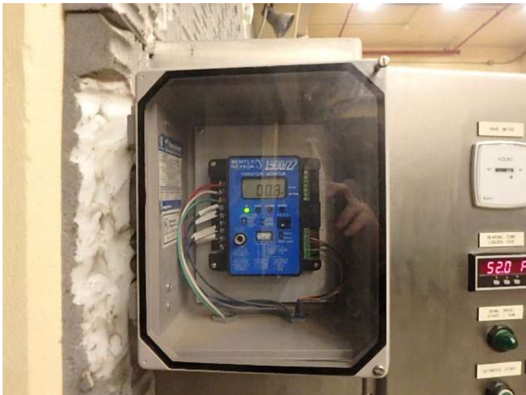
Centrifuge #2 Vibration Monitor
