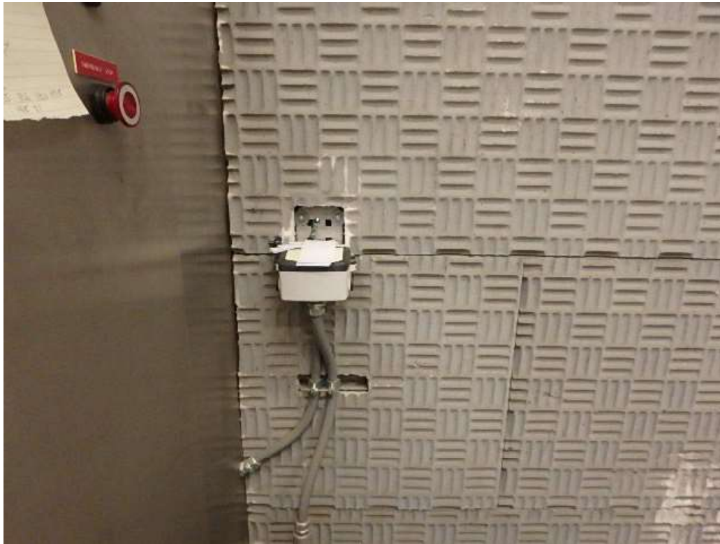
Centrifuge #2 Flowmeter Box Tie In
