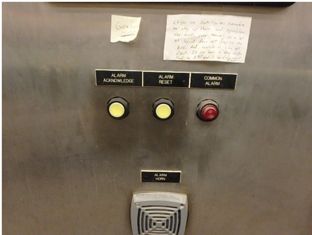
Centrifuge #1 Control Panel Alarms
