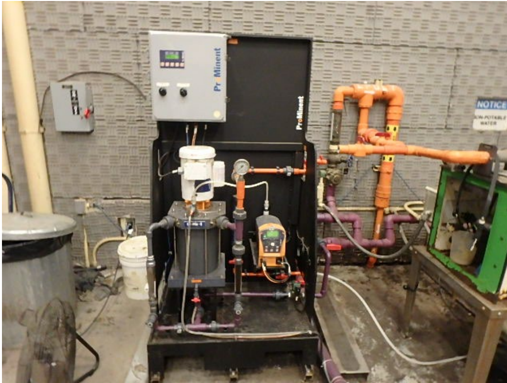
Centrifuge Polymer Injection Example
