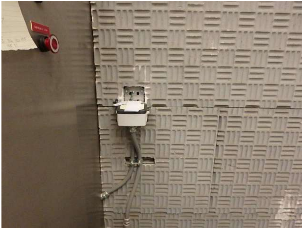
Centrifuge #2 Flowmeter Box Tie In
