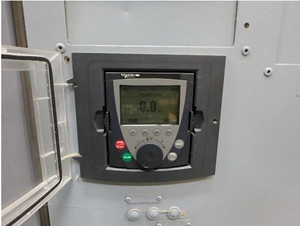
Centrifuge Feed Pump VFD Local Operator Control
