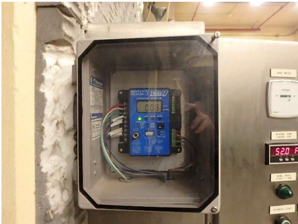
Centrifuge #2 Vibration Monitor
