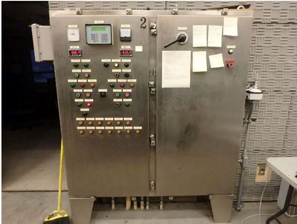
Centrifuge #2 Control Panel
