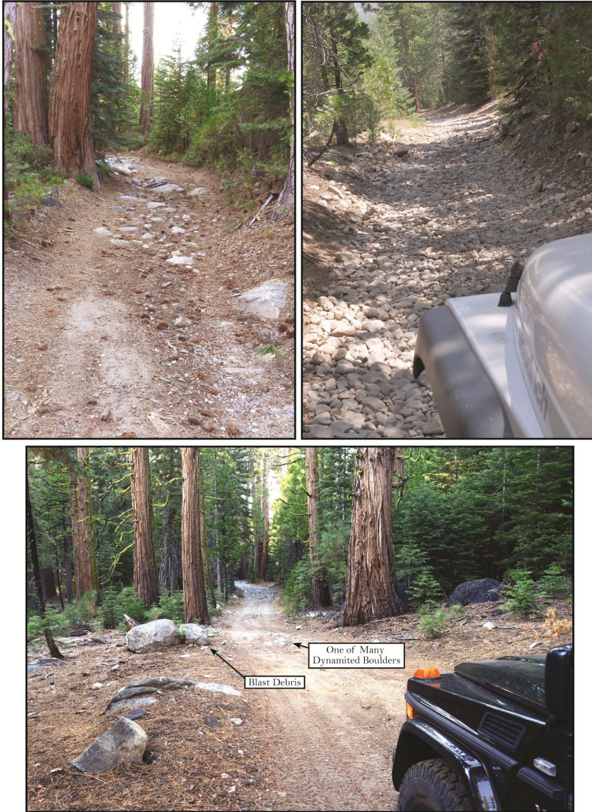
Figure 53. Segment B, Showing Integrity of Original Trail Width and Materials (Courtesy of Harald Pietschmann).
