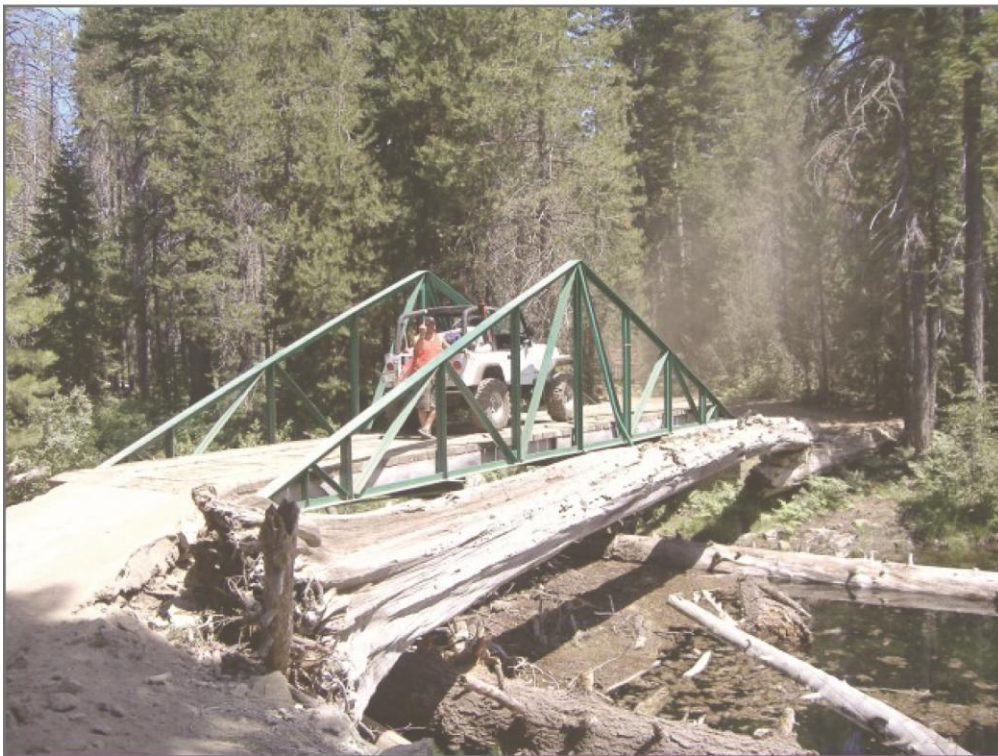
Figure 28. Existing Bridge Over Rubicon River. This steel bridge was constructed by El Dorado County in 1947 and remains today (Pirate 4x4 2012).
