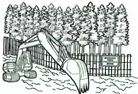
Protective fences should be erected as far out from the trunks as possible in order to protect the root systems.
