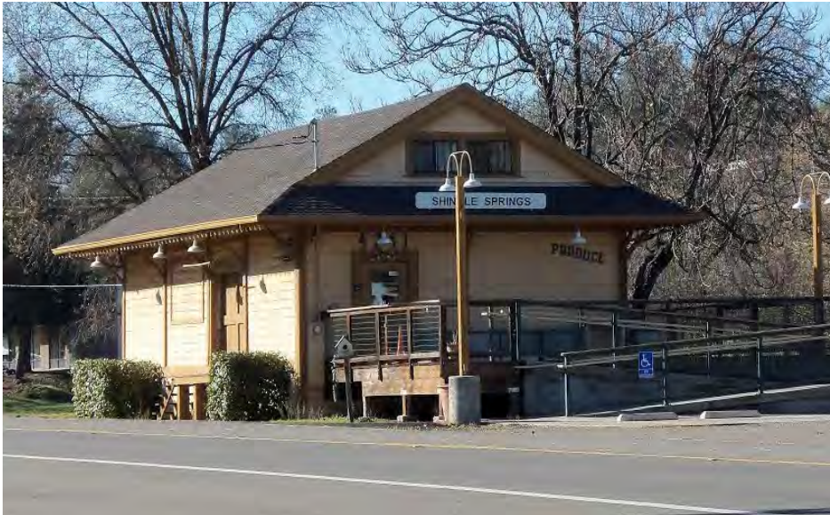
Figure 1: Shingle Springs Railroad Depot (single-story structure)
