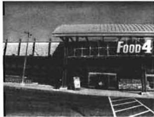
3 West Elevation - Main Entry
