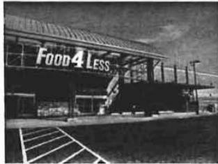
2 West Elevation - Main Entry
