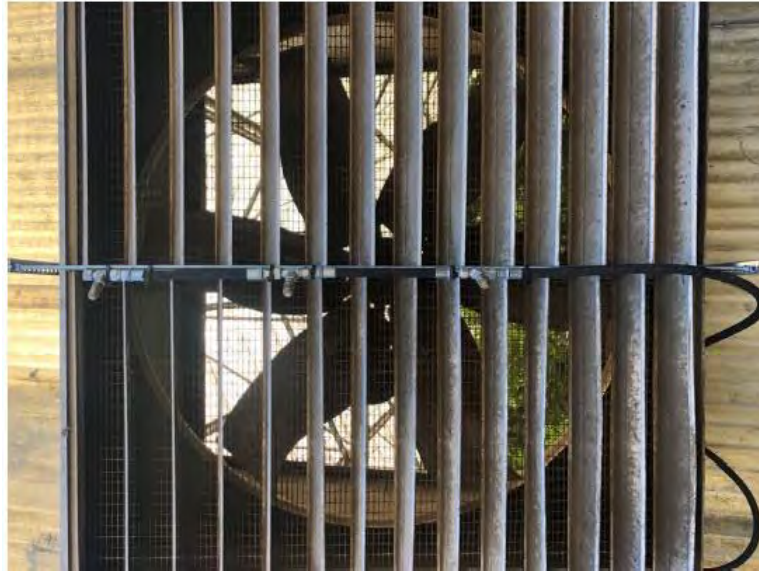
Figure 10 Details of Odor Control Misting Nozzles
