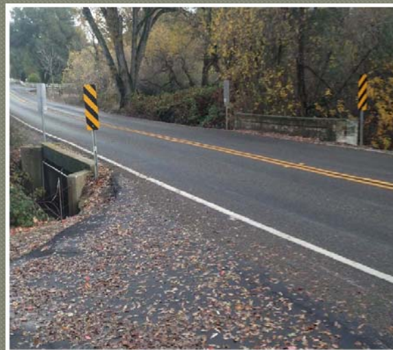
Green Valley Road at Indian Creek Bridge
