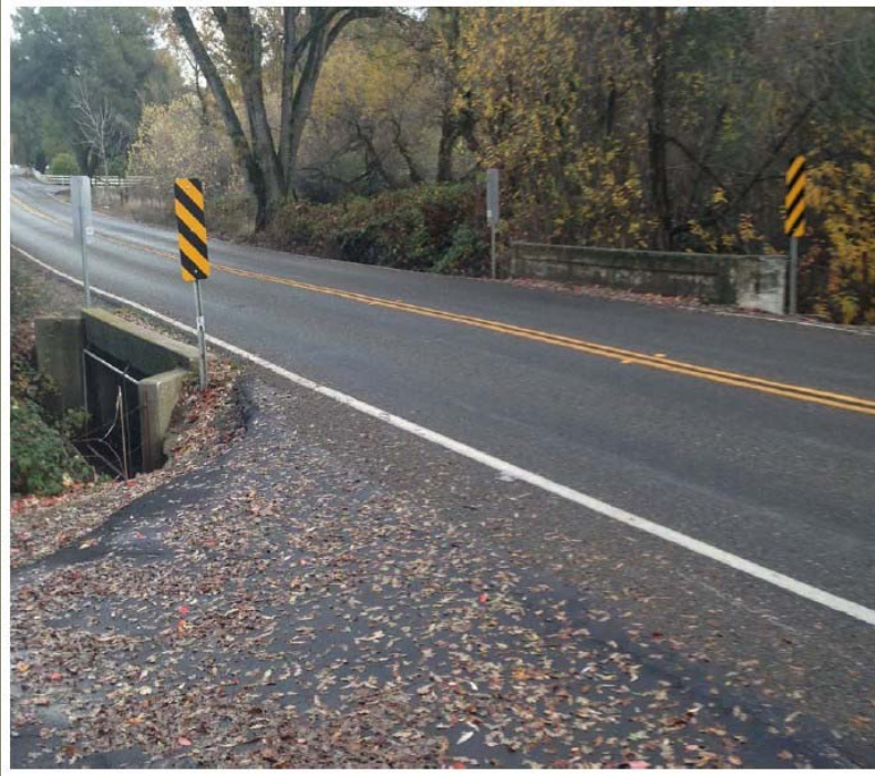
Green Valley Road at Indian Creek Bridge
