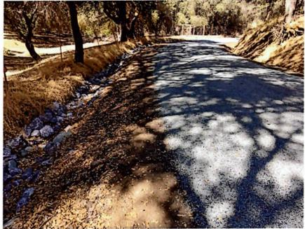
This is a photo you should be very familiar with of one of the chunks of pavement that DOT graded up from the 2006 solid surface of Mt. Murphy Road, and then DOT annually applied dirt and gravel which soon washed away and turned into a potholes/washboard surface:
