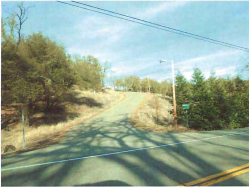
Kaila Way encroachment onto Salmon Falls Road..
