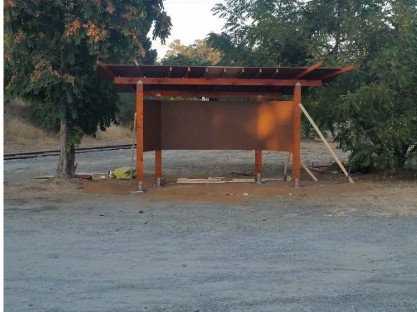
Eagle Scout Project - Kiosk Shingle Springs Depot
