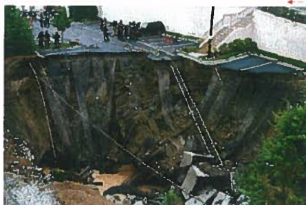
Collapses, such as the sudden formation of sinkholes, may destroy buildings, roads, and utilities.
