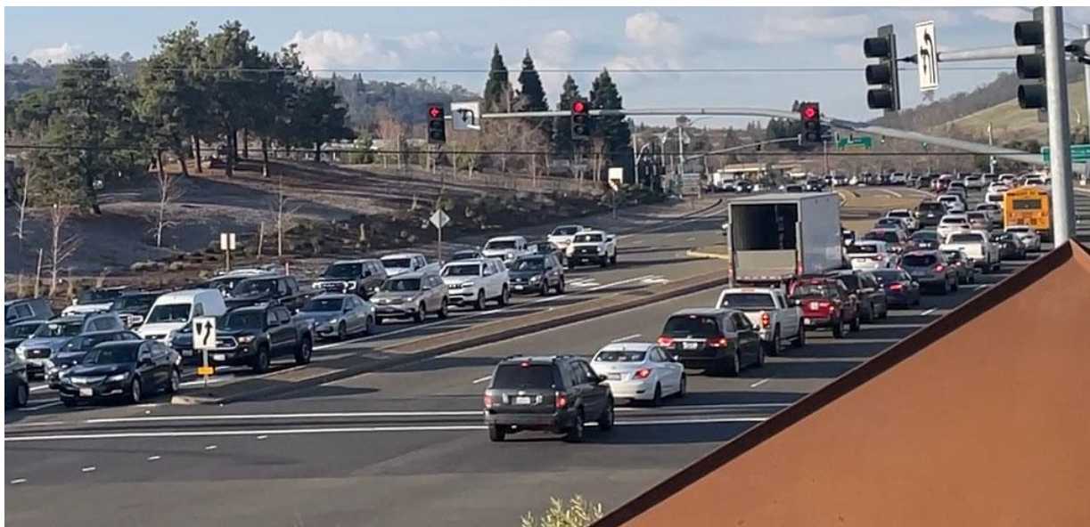
Image 1: An elevated view of Latrobe Road at White Rock Road shows a queue in the third northbound lane spilling back into the intersection during the PM peak hour.
