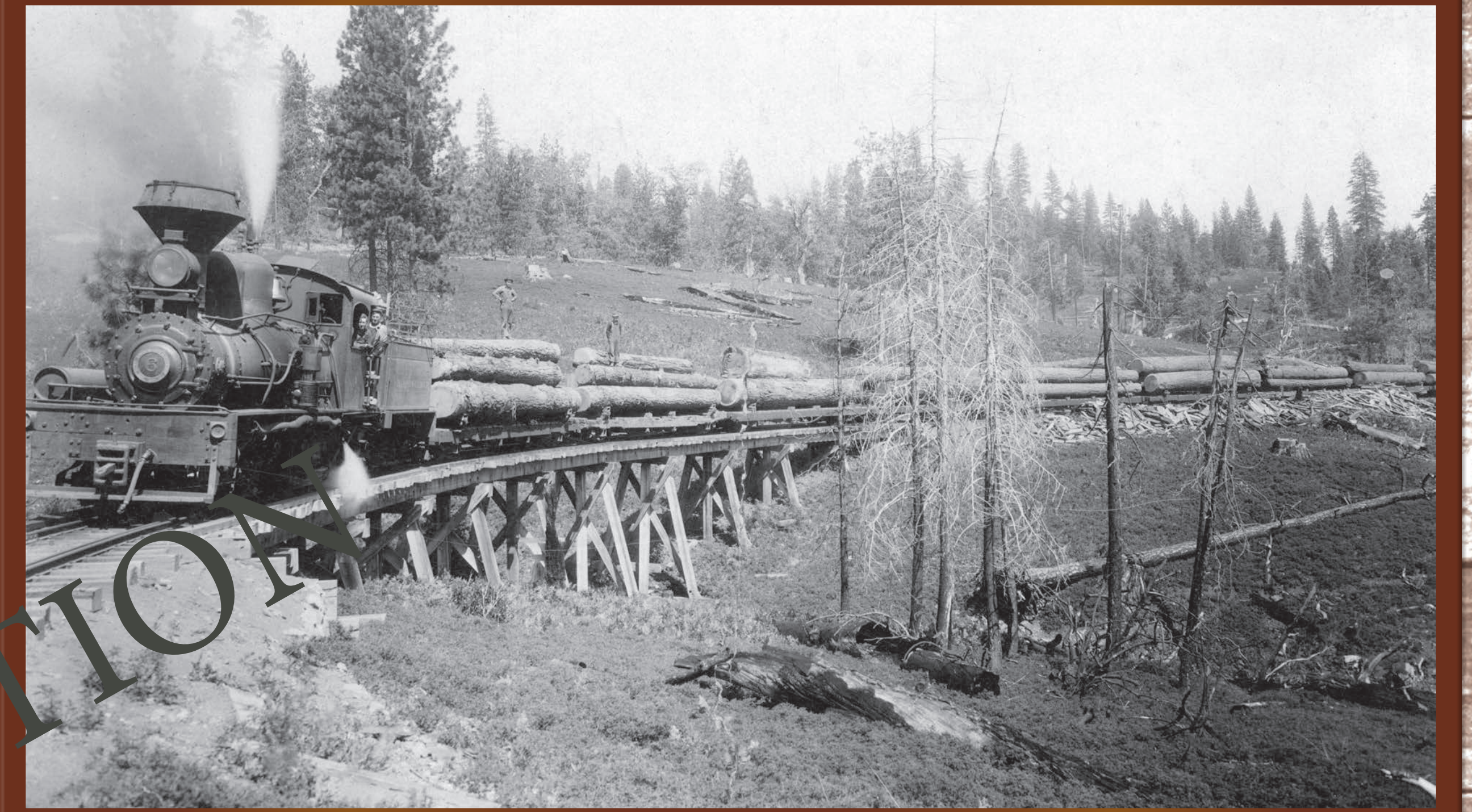
The Caldor Railroad narrow gauge rail carries logs toward Diamond Springs. This narrow gauge track was 3 feet wide, whereas standard gauge track was 4' 8 1/2".
