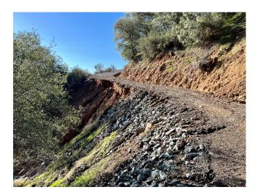
Jurgens Road which is considered "seasonally impassable" is washed out at Weber Creek. The Department has visited the site and determined debris which has washed into what was the road with a height of approximately six feet needs to be removed and the road repaired once waters have receeded.
