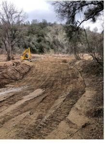
Clear Creek Road experienced a sink hole on one side of the culvert and was repaired the following day. However, the other side of the culvert developed a sink hole and is currently being repaired. The road is closed as of March 14<sup>th</sup> and will be reopened as soon as the repair is completed.
