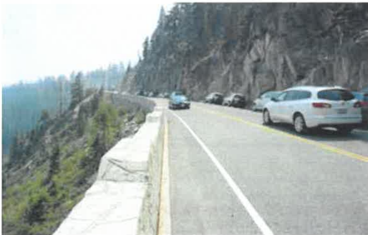
The congestion on the 89 corridor makes emergency response challenging and inefficient.
