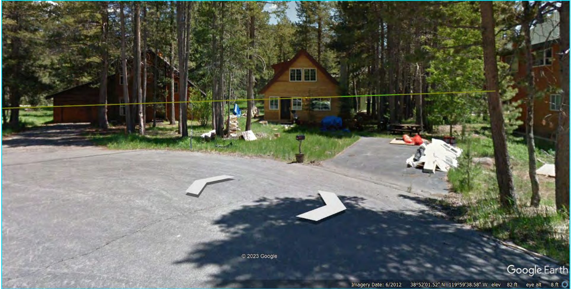
Exhibit F - Existing Conditions
