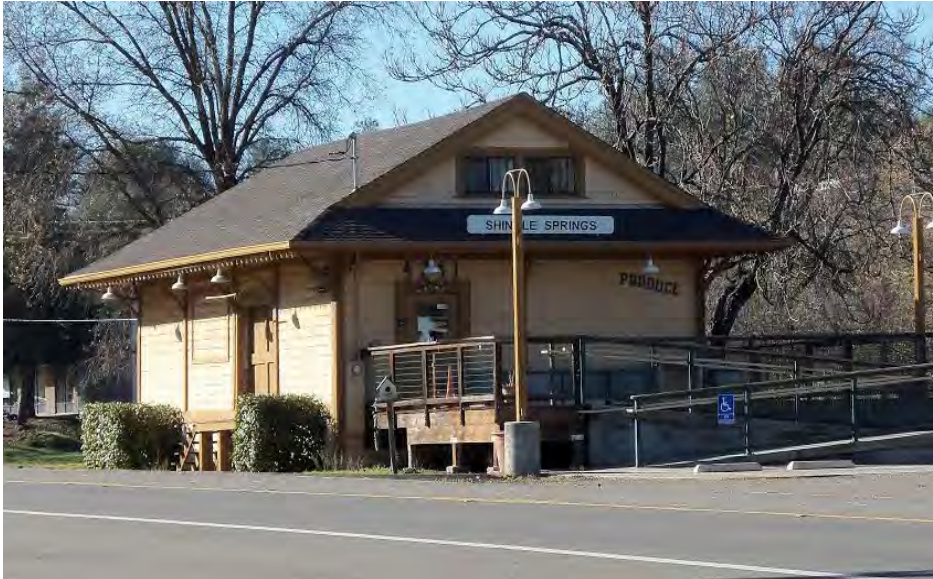
Figure 1: Shingle Springs Railroad Depot (single-story structure)
