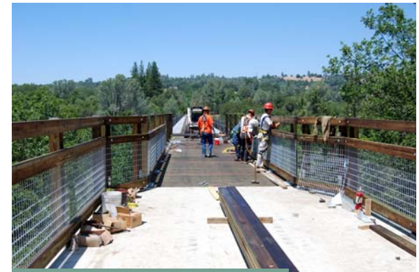
Missouri Flat Trail During Construction 2009
