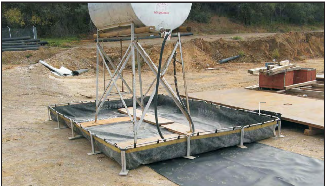
Photo 8: AST with secondary containment. Photo taken 13 November 2007.
