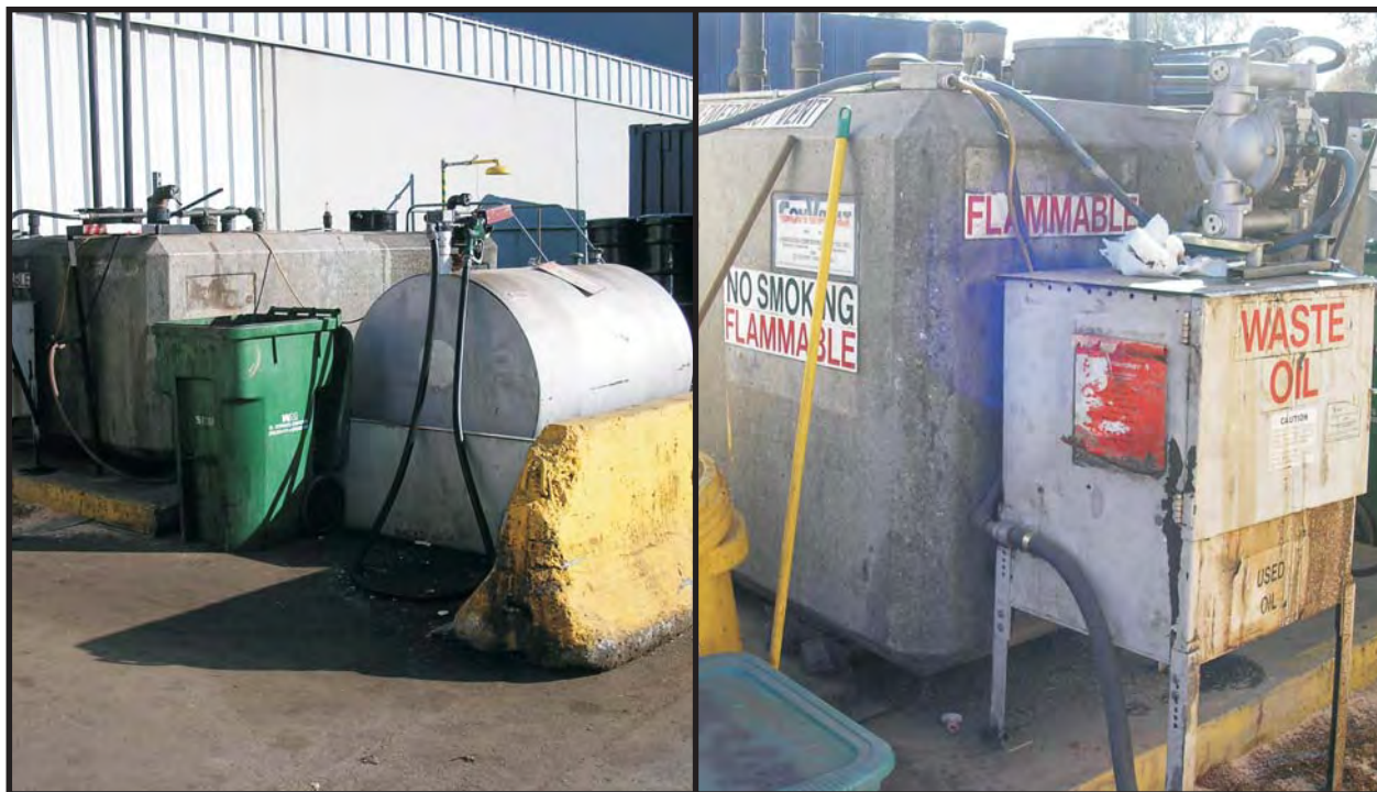
Photo 9: Certified used oil recycling facility outside of the building at the western end of the Waste Connections structure. Waste oil tanks have secondary containment.
