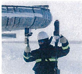
Fig. 2. Pipeline Corrosion Inspection
