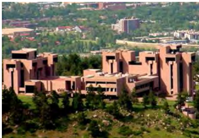
The Mesa Laboratory and Visitors' Center is an Architectural and historical landmark designed by world-renowned architect, I.M. Pei
