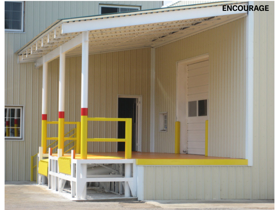
This loading dock's roof screens loading activities from the uses on the second level.
