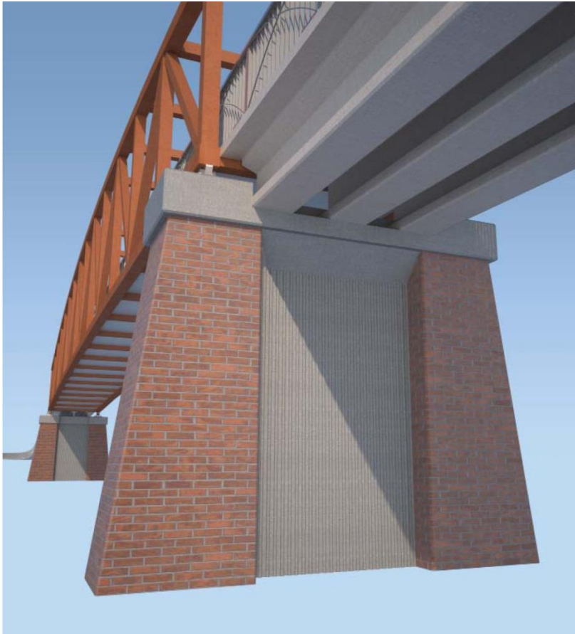
Brick & “Fractured Fin” Concrete Pier
