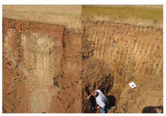
Figure 4-17. Shallow Bedrock with less than 3-Ft of soil cover
