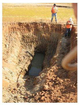
Figure 4-19. Groundwater Found at 6 to 8 Feet in Western Half of Site
