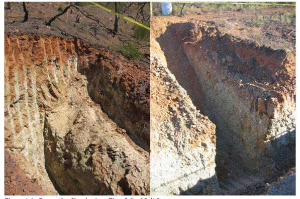
Figure 4-4. Excavation Showing Less Than 3-ft of Soil Cover
