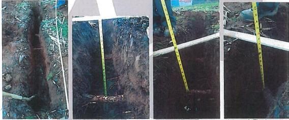
Ten foot long, two-foot deep trench excavated 16 feet from trunk. Two roots were observed. The impact to tree from root pruning of these two roots at this point from the trunk is considered low.
