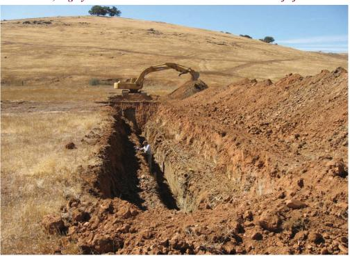
Figure 4-20. Rock not Suitable for Rockfill Embankment, Soil-like in Upper Several feet Across Western two-thirds of Site.
