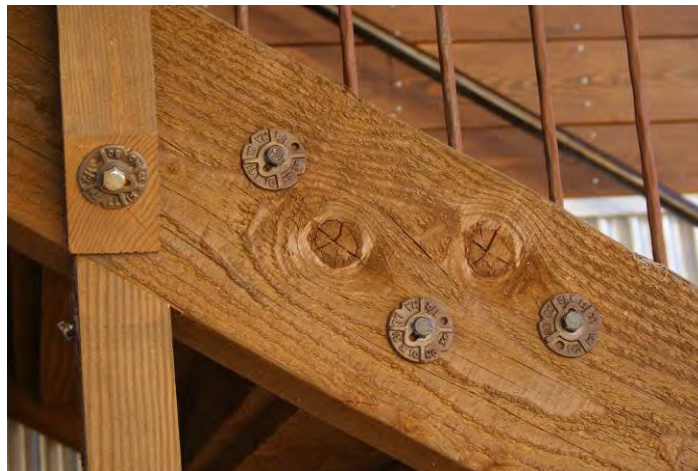
Figure 10 -- Visible Fastenings in Wood Elements at Diamond Center
