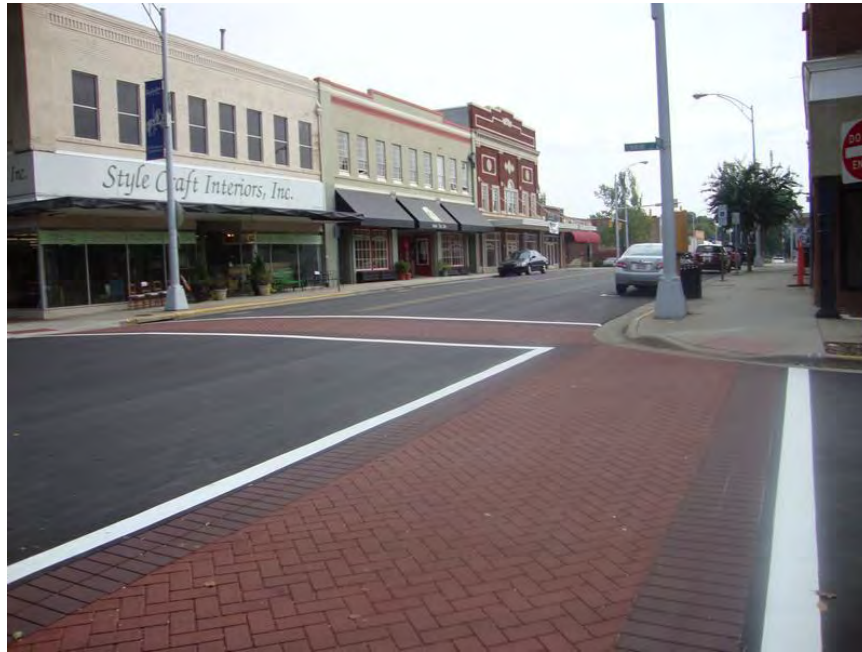
StreetPrint Textured Asphalt Crosswalk, NC
