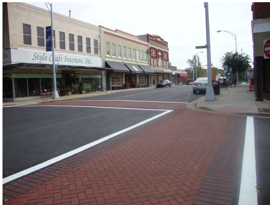
Figure 3 -- StreetPrint Textured Asphalt Crosswalk, NC
