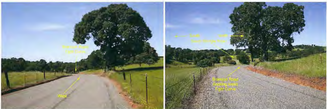
Above: Along Brandon Road, just east of South Shingle Road, exists a very tight, blind curve. Particularly for westbound traffic on Brandon Road, extreme caution must always be exercised when approaching and negotiating this curve. Additional traffic on Brandon Road will certainly exacerbate traffic risks at this location. May 3, 2017.
