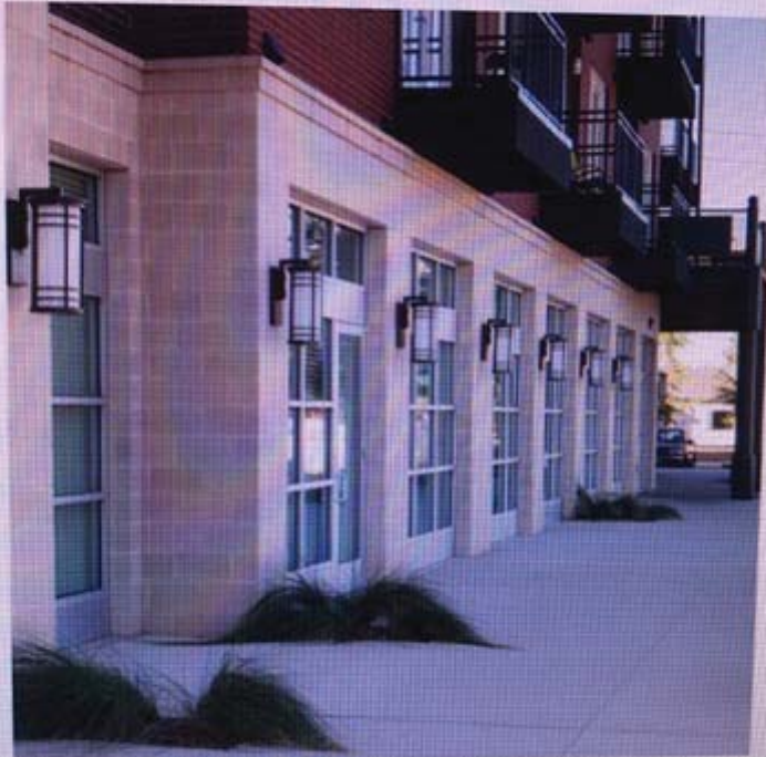
Solid materials, tall ceilings, frequent pilasters, divided glazing systems, special light fixtures, and a covered facade articulate spaces that can be either retail or residential. (JHP)
