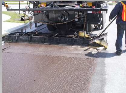
Slurry Seal PCI: 80 – 55 Cost: $28,500/mile
