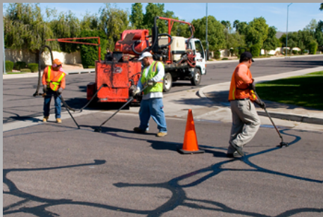
Crack Seal PCI: 90 – 65 Cost: $18,500/mile
