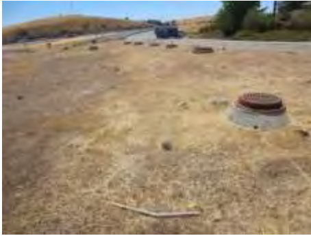
UTILITIES ON SUBJECT PROPERTY LOOKING SOUTHWEST
