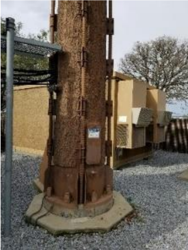
Photos of Structural Bracing on the existing SBA Tower:
