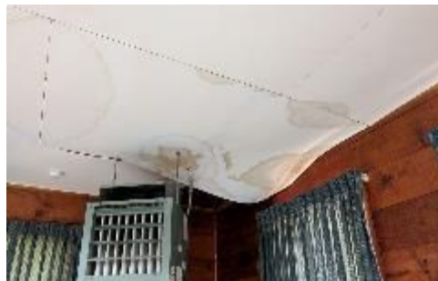
An example of damage to the interior due to roof leaks.
