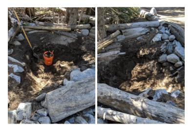
4. The Loon Lake Intertie #2 segment from the Whale Bones to the Intertie with the Rubicon Trail. This segment was adopted by Auburn Jeep Club. This segment also has granite slabs that were treated with Bio Response for spills. 36 five gallon buckets that equate to .90 cubic yards of sediment were removed from this segment.
